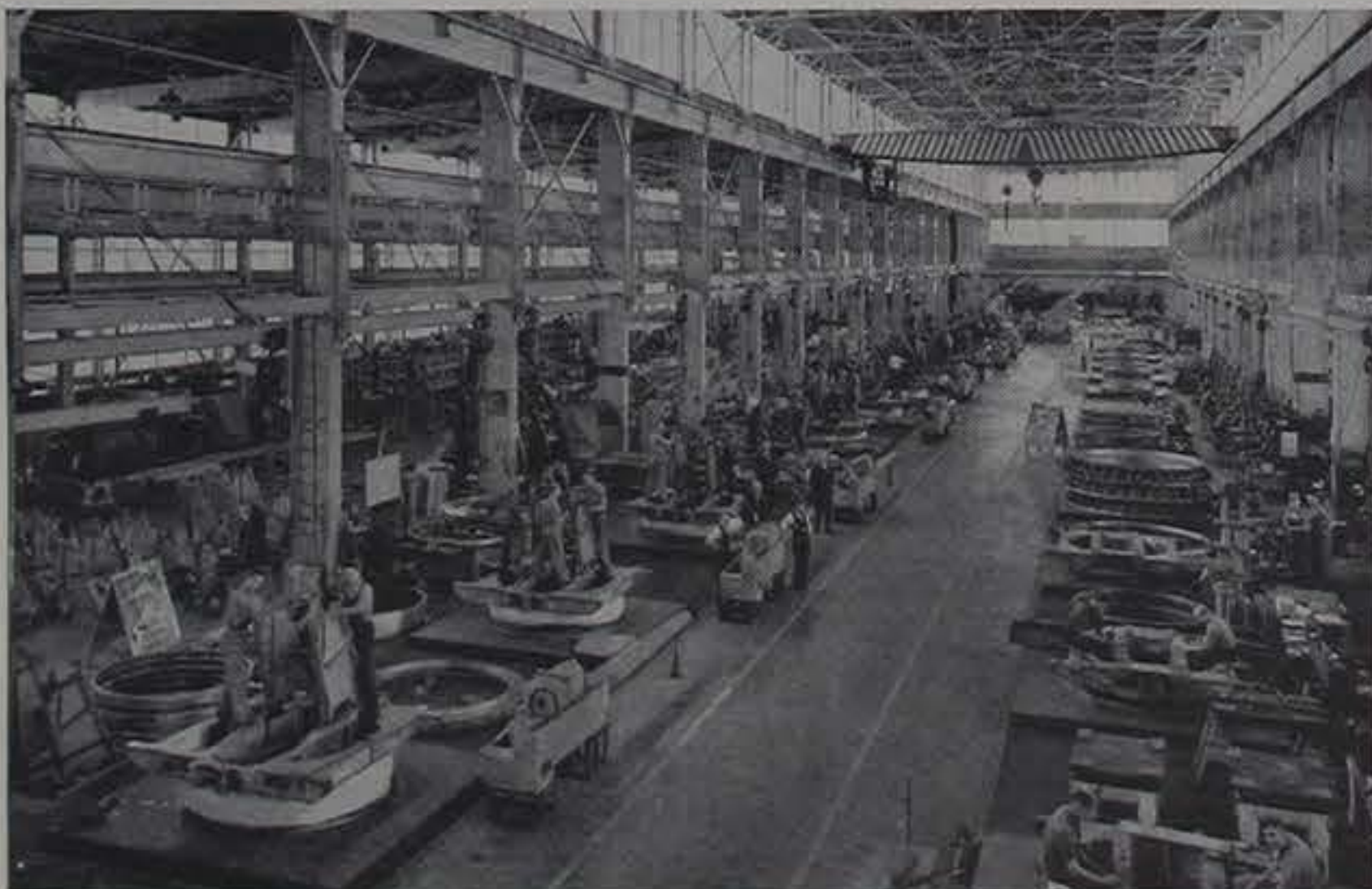
Part of the plant operating "two months ahead of the unbelievable."
